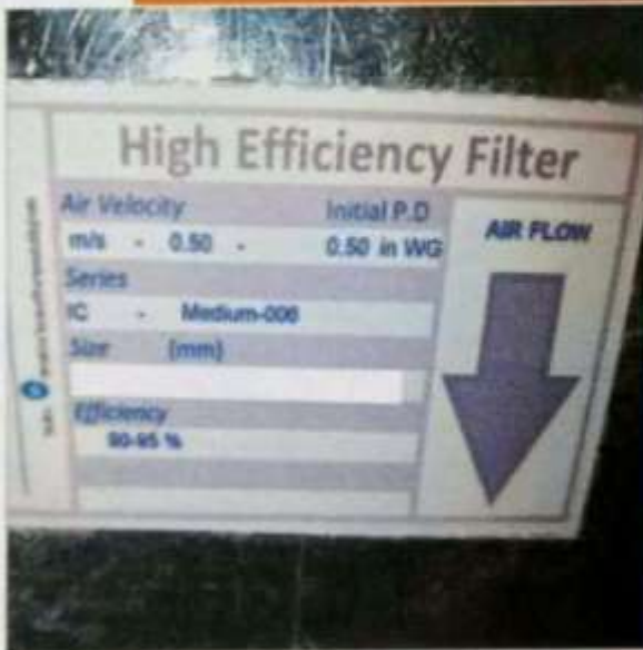
HEPA Filters for HVAC System (Size: 480 mm x 810 mm x 100 mm) L 480 mm x W 810 mm x D 100 mm
